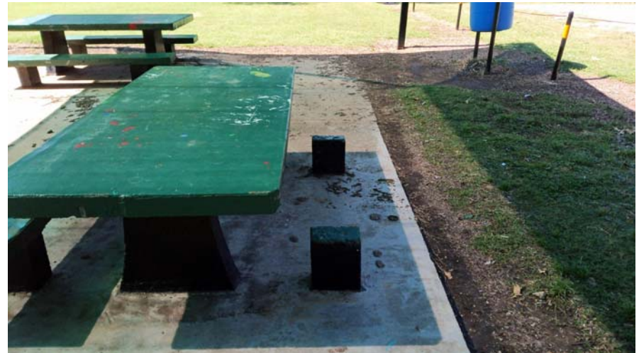
One bench on this concrete picnic table has been broken and is due for replacement.
