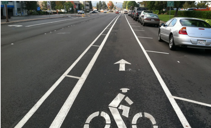
Bike Lanes are on-street facilities designated for bicyclists using stripes and stencils. Bike lanes may include buffer striping to provide greater separation between bicyclists and parked or moving vehicles. Bike lanes are the preferred treatment for all arterial and collector streets on the bikeway network, and not typically installed on low-volume, low-speed residential streets.
