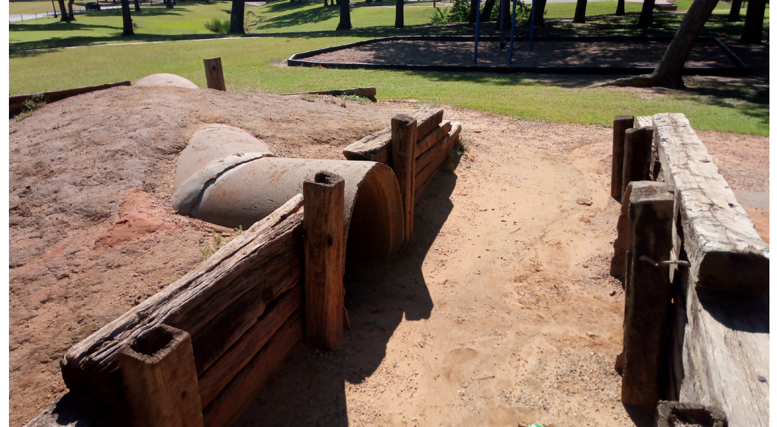
A play structure built from timbers and stormwater pipe. The wooden components are significantly weathered and splintering.
