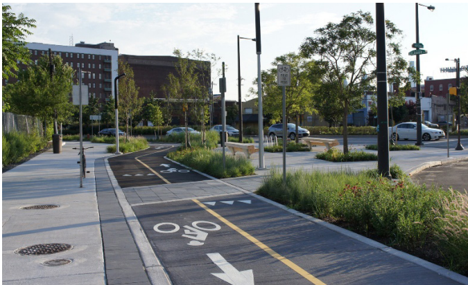
Protected Bike Lanes provide space that is exclusively for bicyclists and separated from motor vehicle travel lanes, parking lanes, and sidewalks. Parked cars, curbs, bollards, or planter boxes provide physical separation between bicyclists and moving cars.
