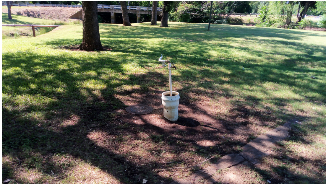
A drinking fountain build from a section of pipe filled with concrete.
